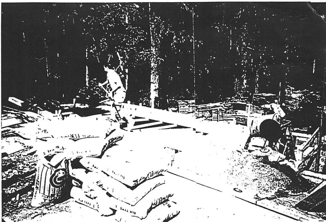
Right: Building 1 Foundations. Otmar Heimbucher mixes and Walter Marks and Joe Watanabe place mixed concrete for footings to support the lounge and kitchen building.
